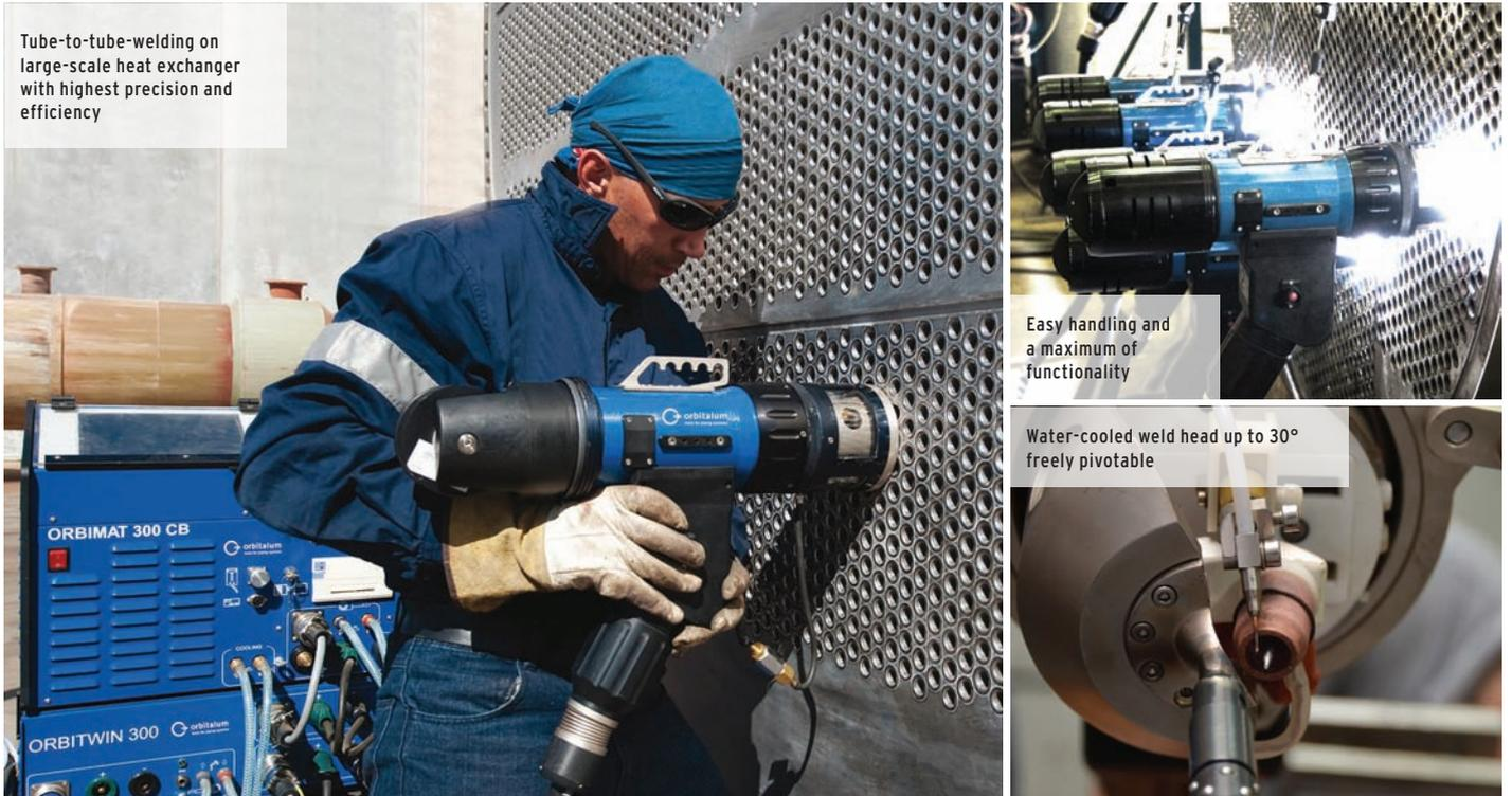
Tube-to-tube-welding on large-scale heat exchanger with highest precision and efficiency
